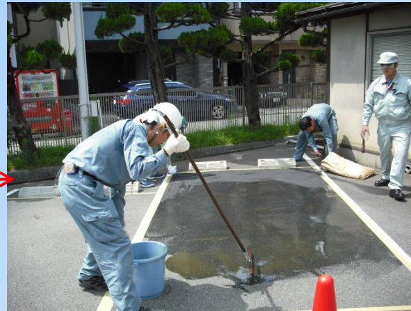
Base resin (Prime coating)
