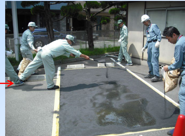
Distributing Icetool aggregate
