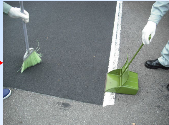
Excessive aggregate must be swept away
