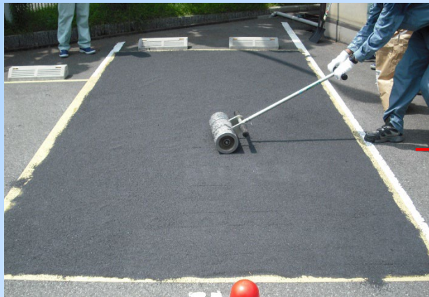
Roller compacting
