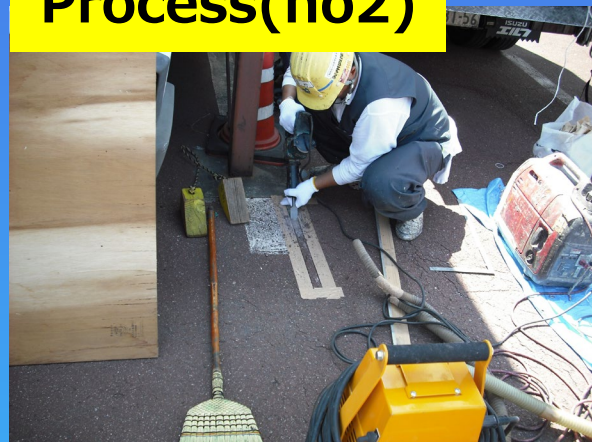
① Cutting the part by a handy type of road cutter
