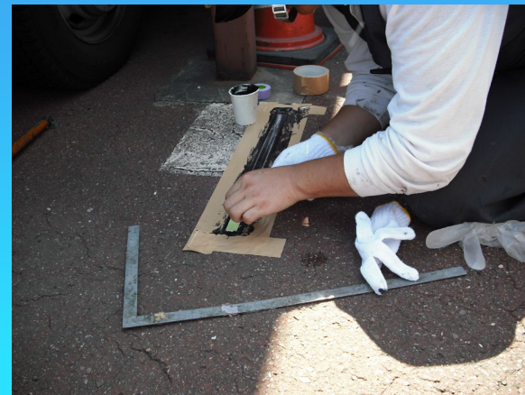
④ Peeling the cover seal material off
