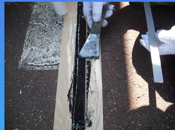
② pouring and pasting resin
