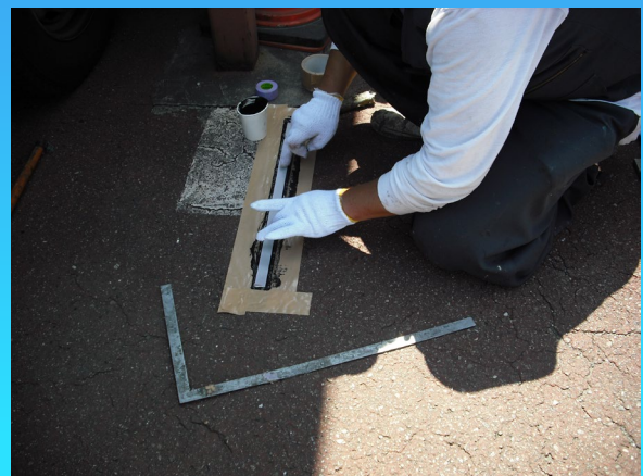
③ Installing Lumo Line
