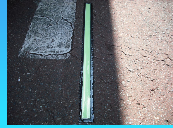
② pouring and pasting resin
